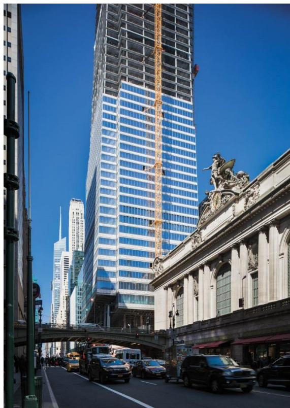
Towering over Grand Central Terminal, One Vanderbilt is the tallest office building in midtown Manhattan. Cognizant of the building's prominence, architecture firm KPF designed terra-cotta spandrels that zigzag up the 1,400-foot-tall skyscraper.
