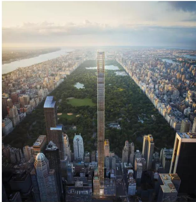
The building overlooks Central Park (HayesDavidson)
