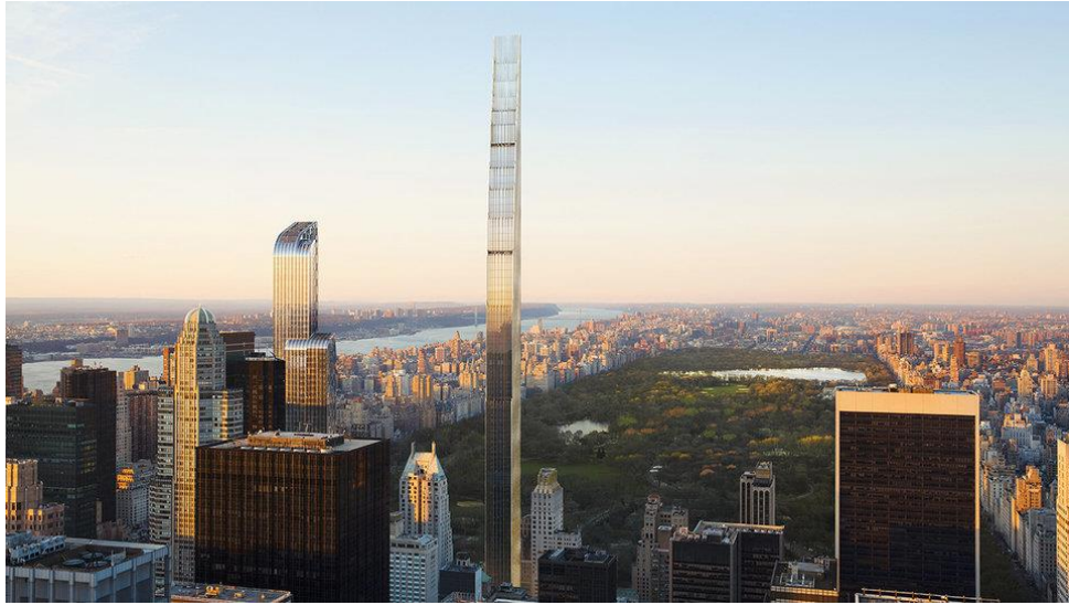
The project is scheduled to be completed in 2020
