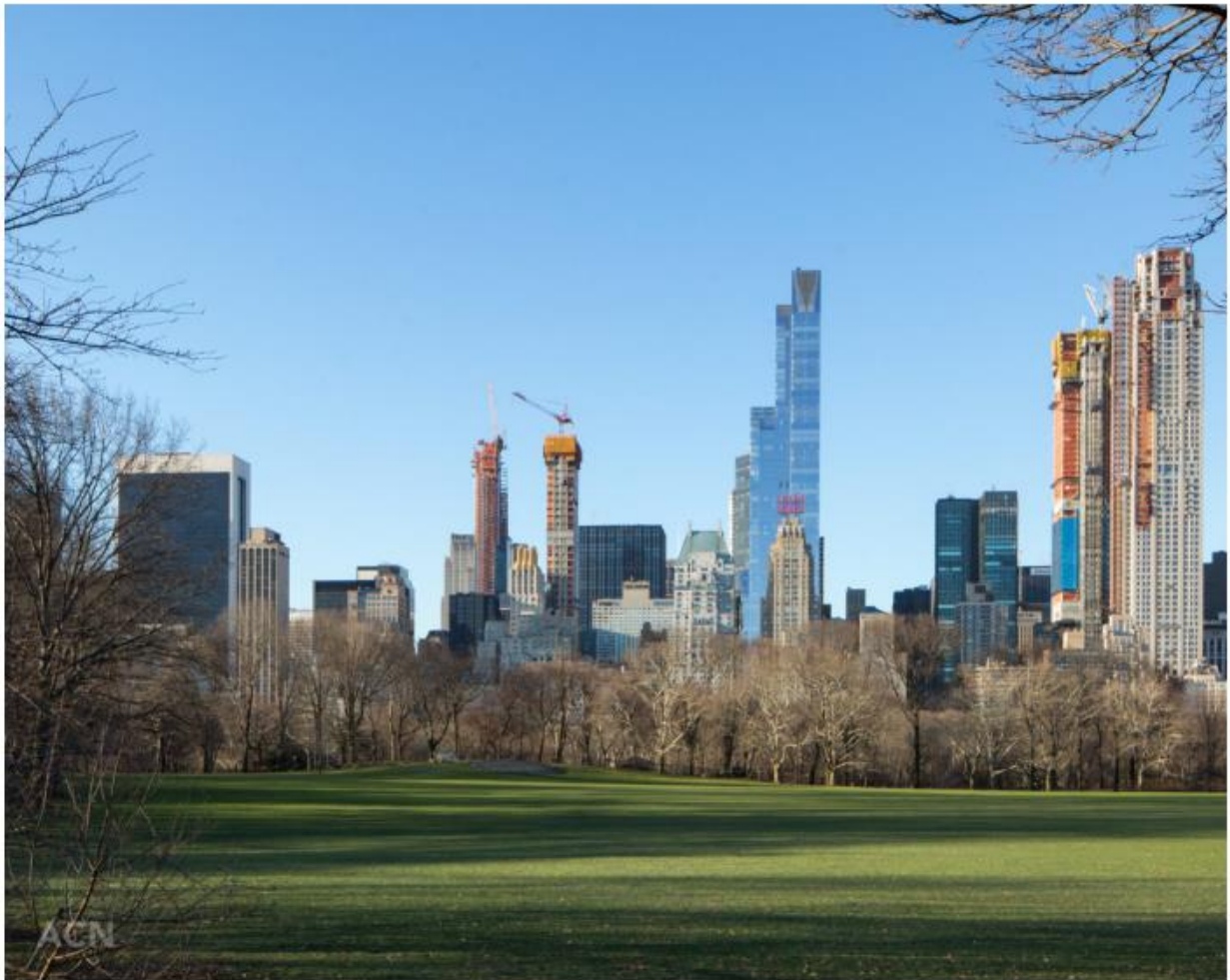
Under construction 55w53 (left) and 111 West 57th Street (right) from across Sheep Meadow, image captured in March, by Andrew Campbell Nelson
